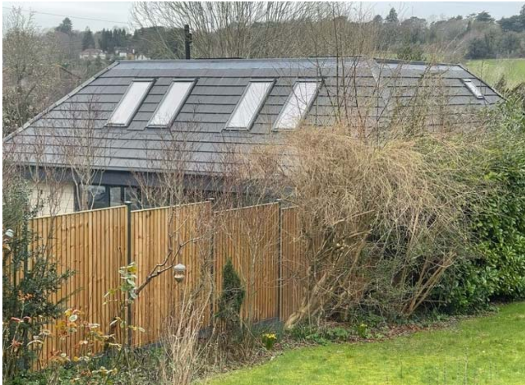
Figure 9 – Photo of outbuilding from rear of No.98 Downs Road
