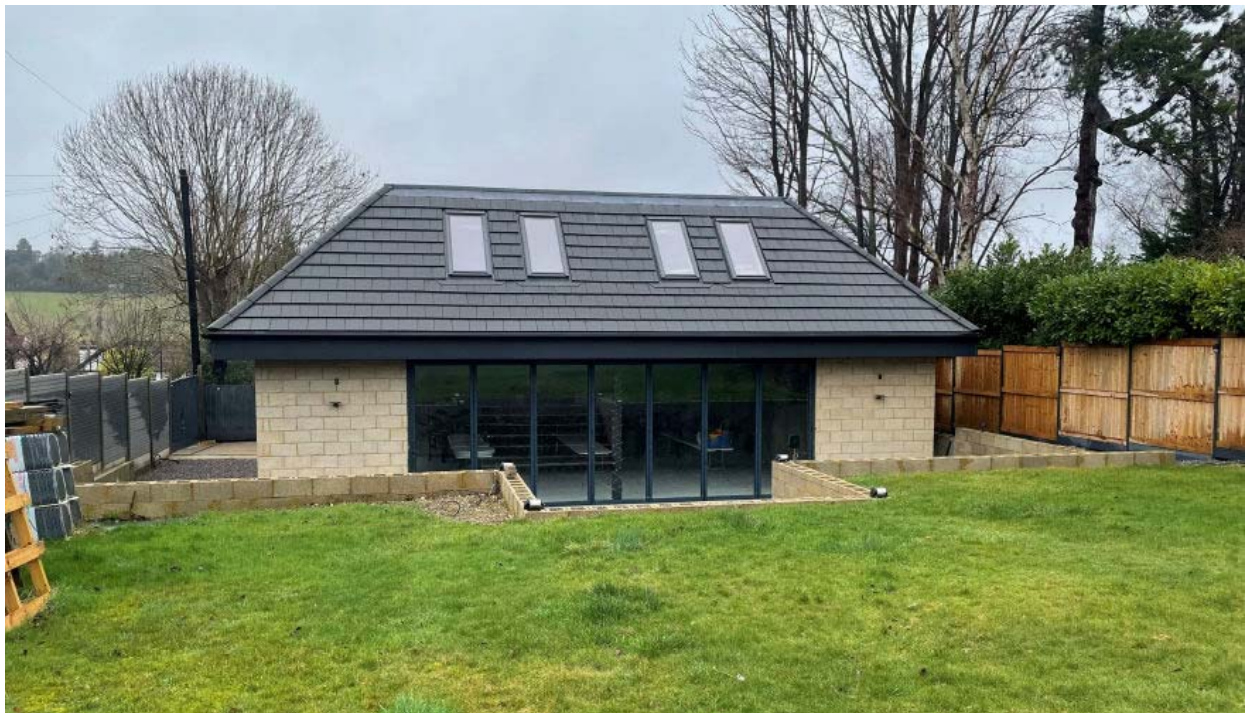
Figure 5 – Photo of outbuilding as built from rear garden of 100 Downs Road
